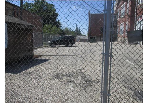
Erosion is evident in the asphalt of the courtyard. The parking spaces can be replaced with porous pavement to capture, treat, and infiltrate roof and pavement runoff. A preliminary soil assessment suggests that the soils have suitable drainage characteristics for green infrastructure.
