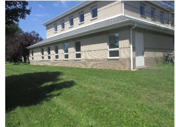
Downspouts originating from the roofs of the two buildings can be disconnected and rerouted to two rain gardens to capture, treat, and infiltrate roof runoff. A preliminary soil assessment suggests that the soils have suitable drainage characteristics for green infrastructure.
