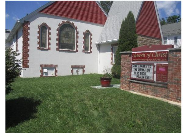
Existing downspouts from the roof can be disconnected and rerouted to a rain garden near the front of the church, which will capture, treat, and infiltrate roof runoff. A preliminary soil assessment suggests that the soils have suitable drainage characteristics for green infrastructure.
